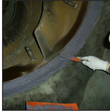
Belzona ® 1812 being applied
