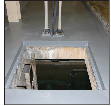
Rebuilt, protected, a first class job
