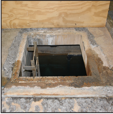
Floor prepared for resurfacing
