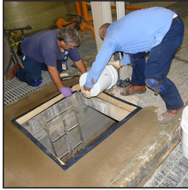
Reshaping the access opening
