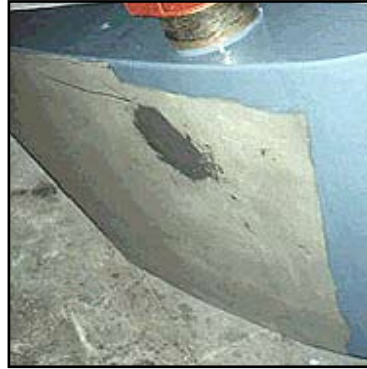
Rebuilding cavitation damage.
