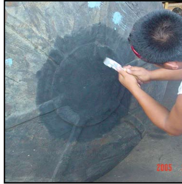
Surface preparation for the fender.
