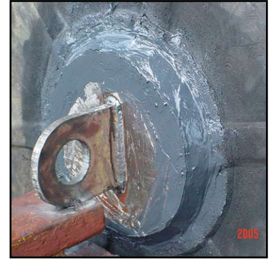
Finished application - metal lifting device is attached to the fender.
